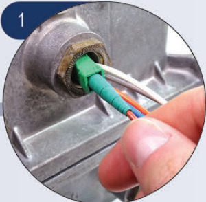
1 Feed connectors through node entry port
